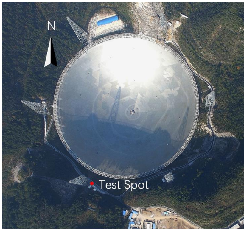
Fig.1 RFI test spot at the bottom of the 7H feed support tower.
